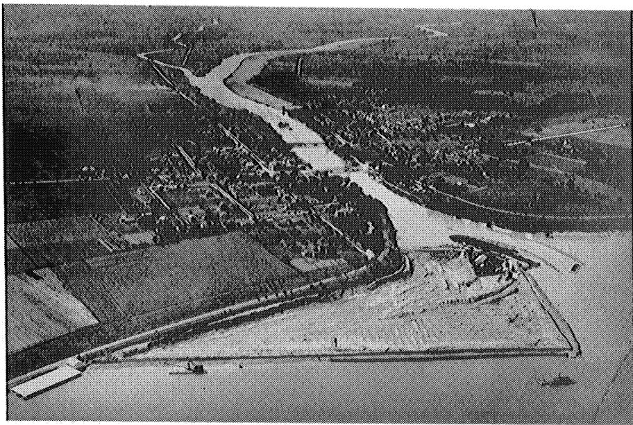
Entrance to Welland River section of power canal, showing intake works under construction and village of Chippawa.
